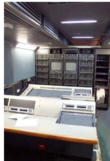
Internal View looking backwards towards the Engineering Section
