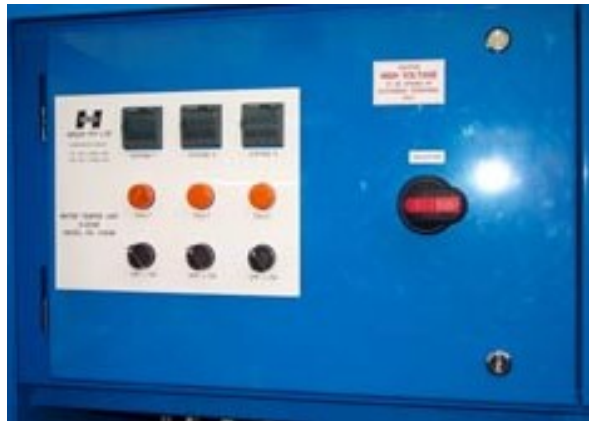
Typical Control Panel for a 3 Zone Unit
